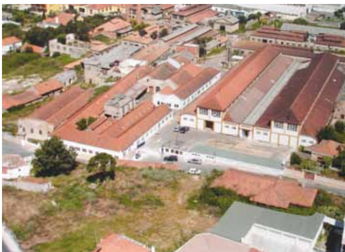
Aerial Plant View
